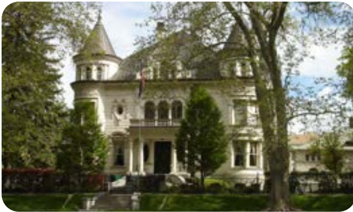
Kearns Mansion/Utah Governor's Mansion Roof and Window Restoration
