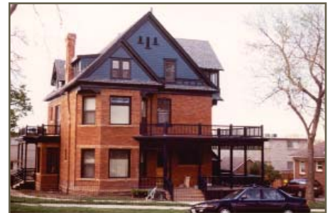
Avenues home after rehabilitation, Salt Lake City
